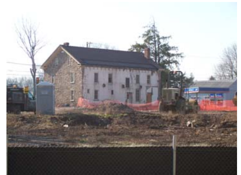
Renovation work begins on the Audubon Inn
